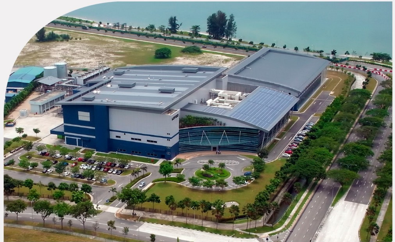
Lonza contract manufacturing facility in Singapore
