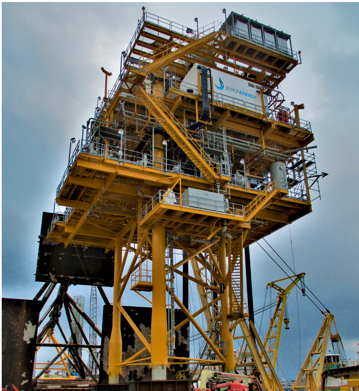
Tripod platform structure for the Byron operated SM 71 field, currently in Galveston, TX to be installed at SM 71.
