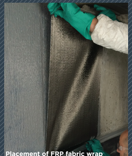
Placement of FRP fabric wrap
