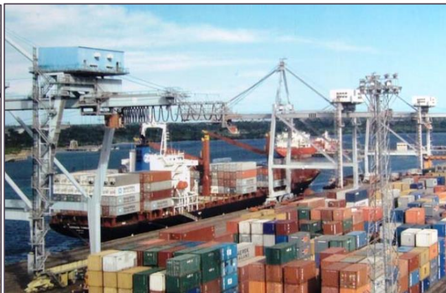
Figure 11: Dar es Salaam Port Container Loading Area
