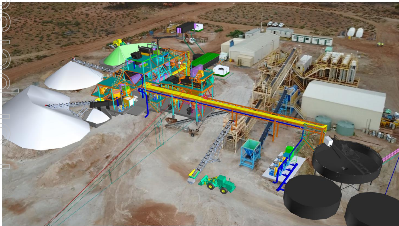
Figure 4: DMS Plant Layout with the existing Tantalum Plant (Provided by Primero)
