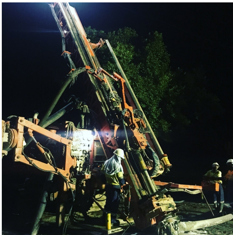
Fig. 2 Drilling operations at Gbane
