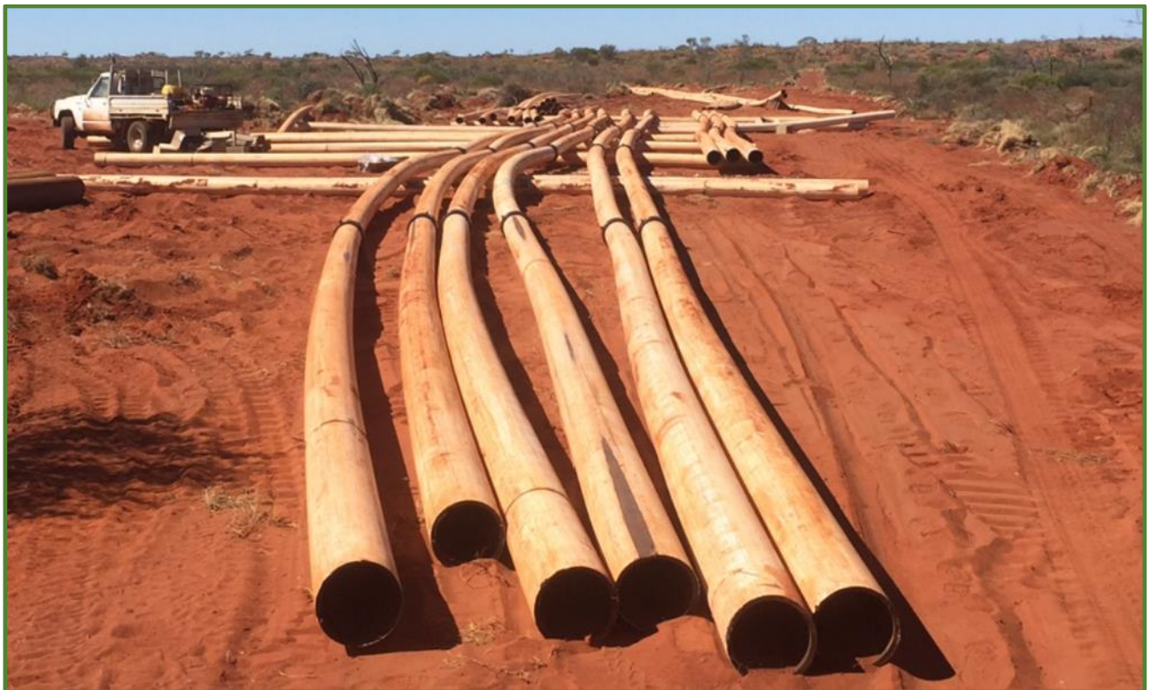
Pipeline assembly area at 10 Mile
