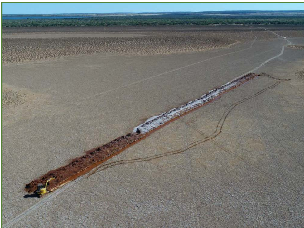
Aerial view of 10 Mile trench installation
