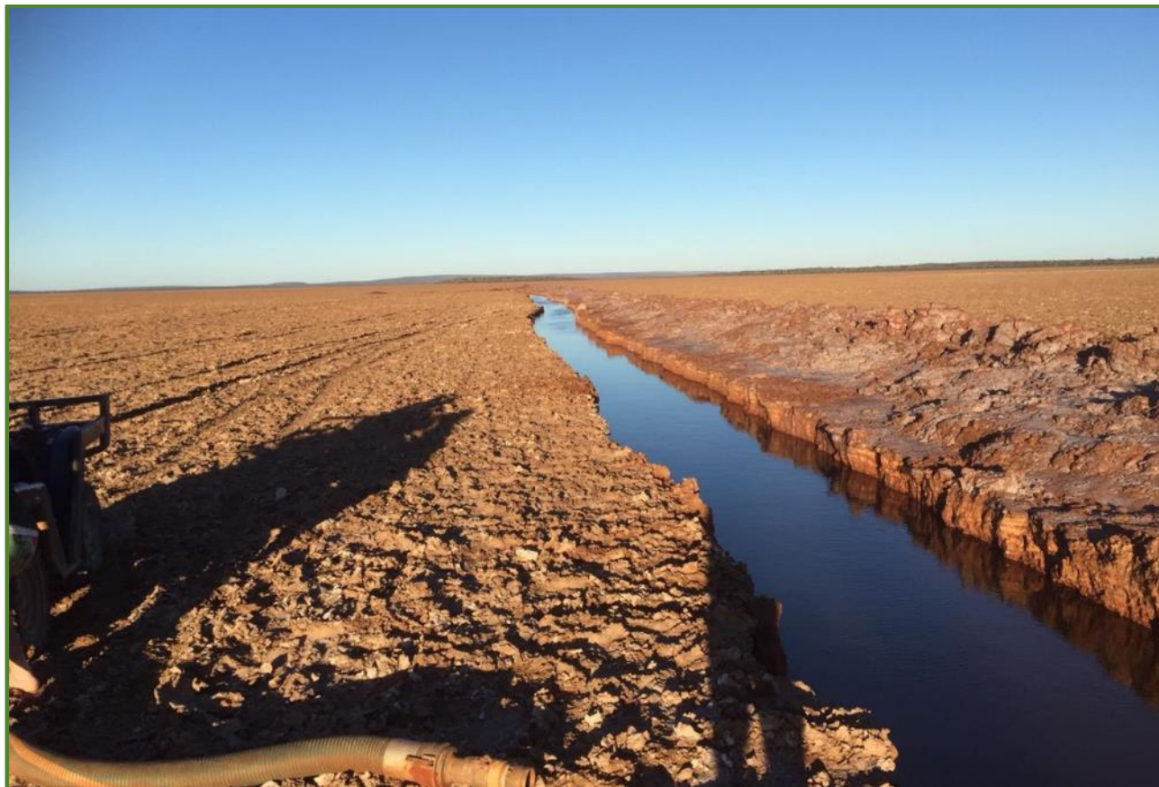
Trench installed at 10 Mile
