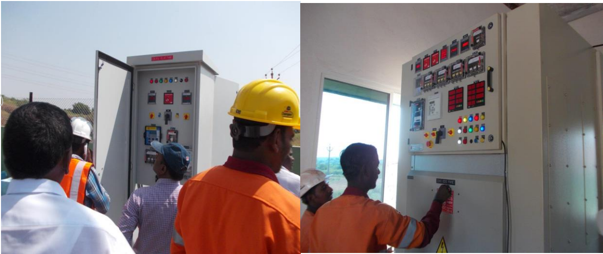
33kV Vacuum Circuit Breaker (VCB) Panel powered up
