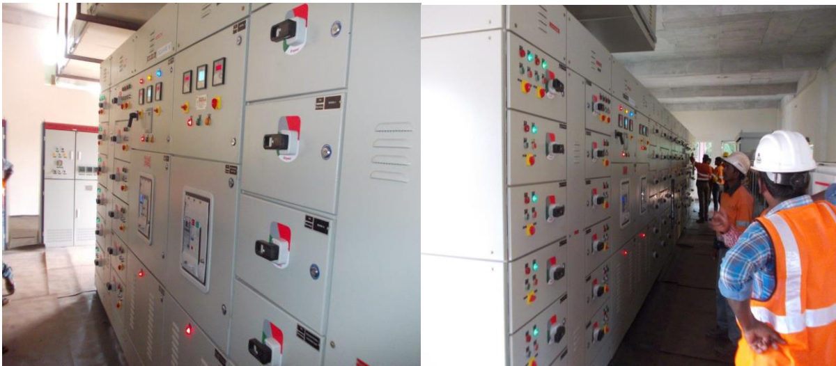
33kV Vacuum Circuit Breaker (VCB) Panel powered up
