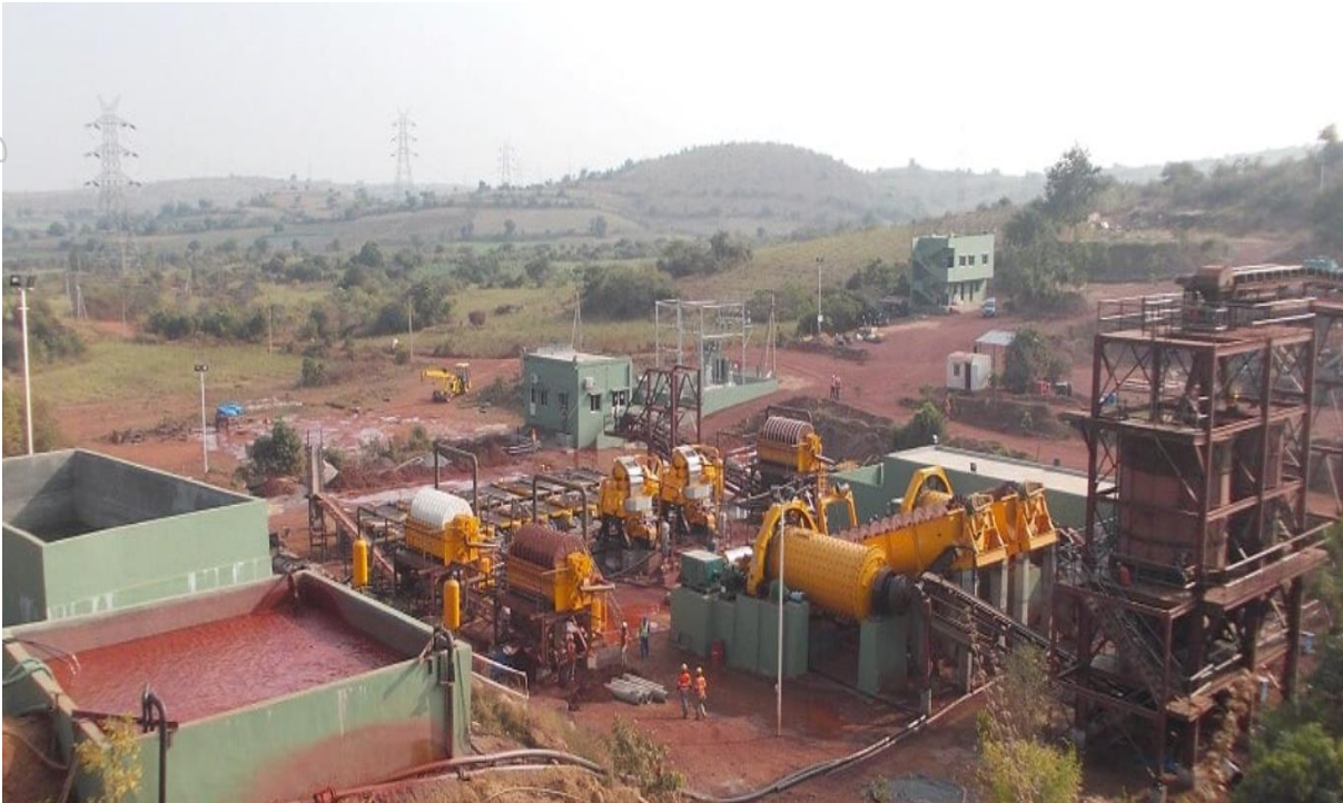
Wet plant overview
