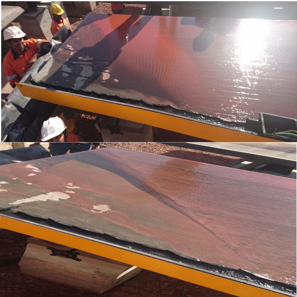
Density Separation Equipment Commissioning
