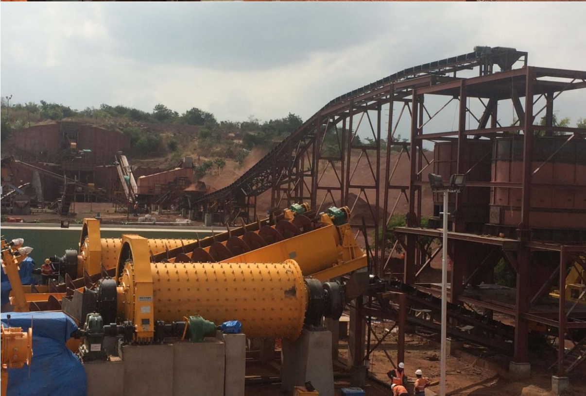
Plant being loaded with first iron ore
