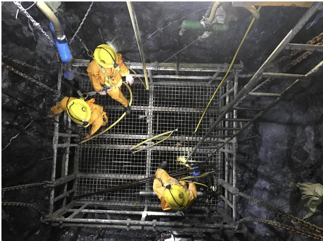
Picture 1: E15 sinking stage lower deck, on the bench
