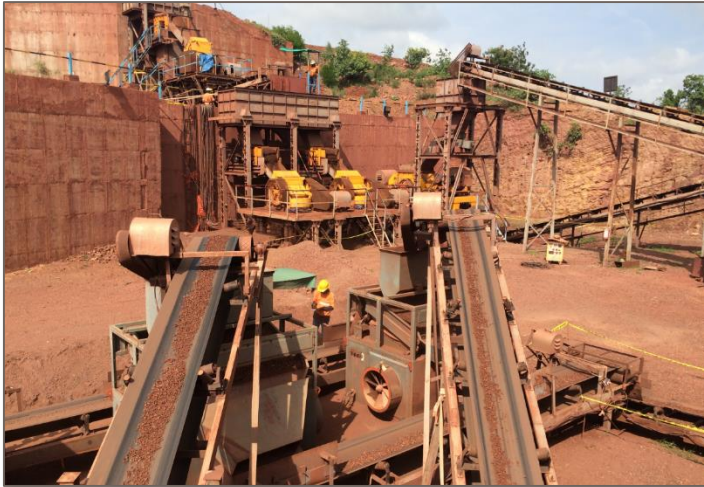
Kurnool beneficiation plant, Phase 1 production
