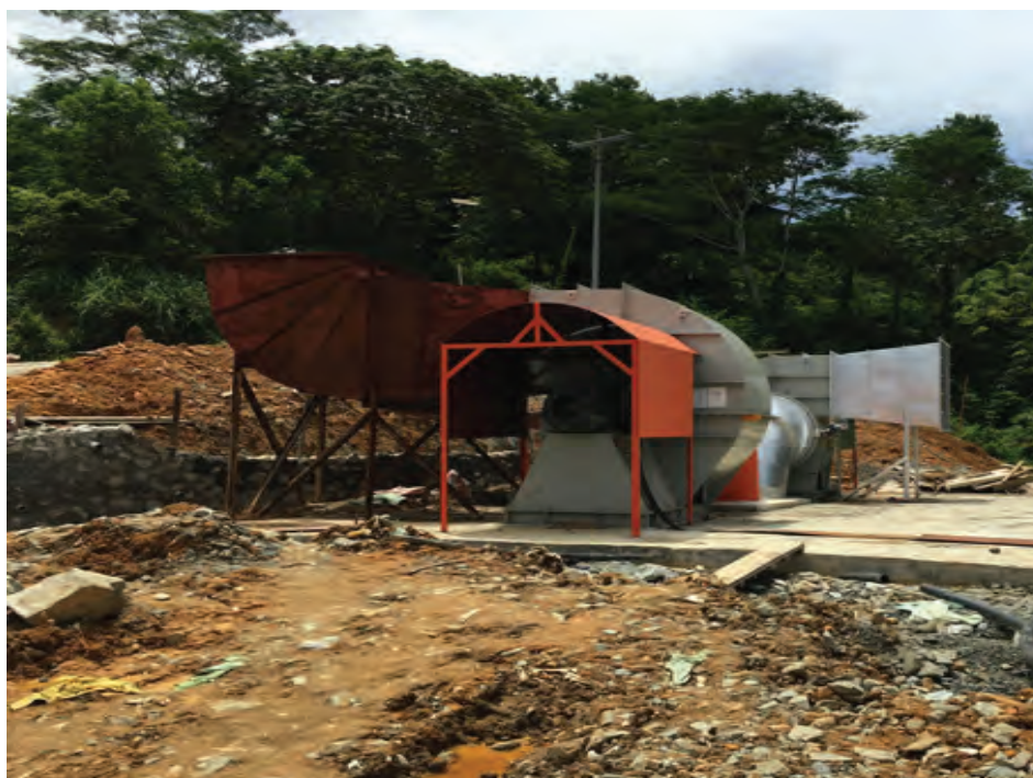
Picture 5: The 2 new Centrifugal Fans before commissioning
