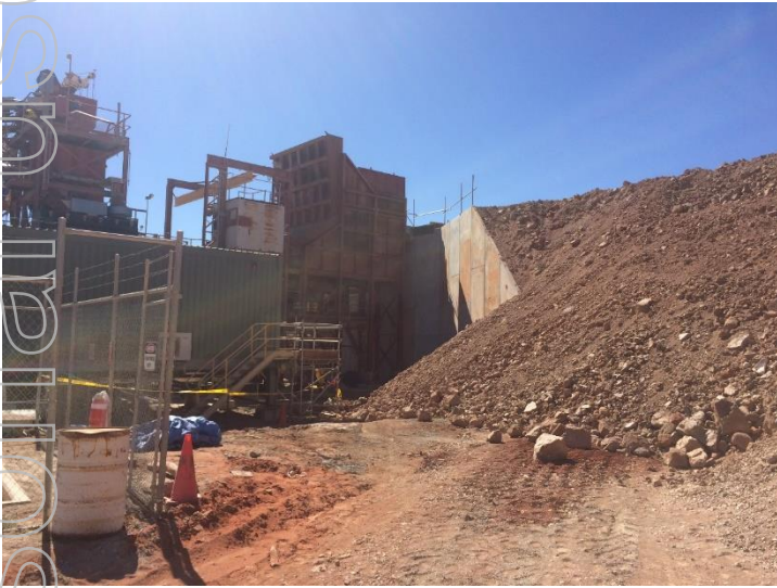
Photo 4: ROM wall constructed and backfilled
