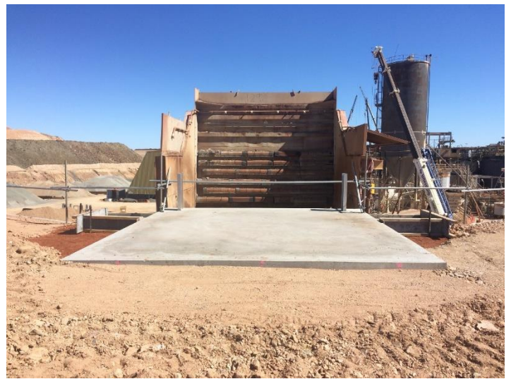
Photo 5: Concrete Pad at the Primary Crusher
