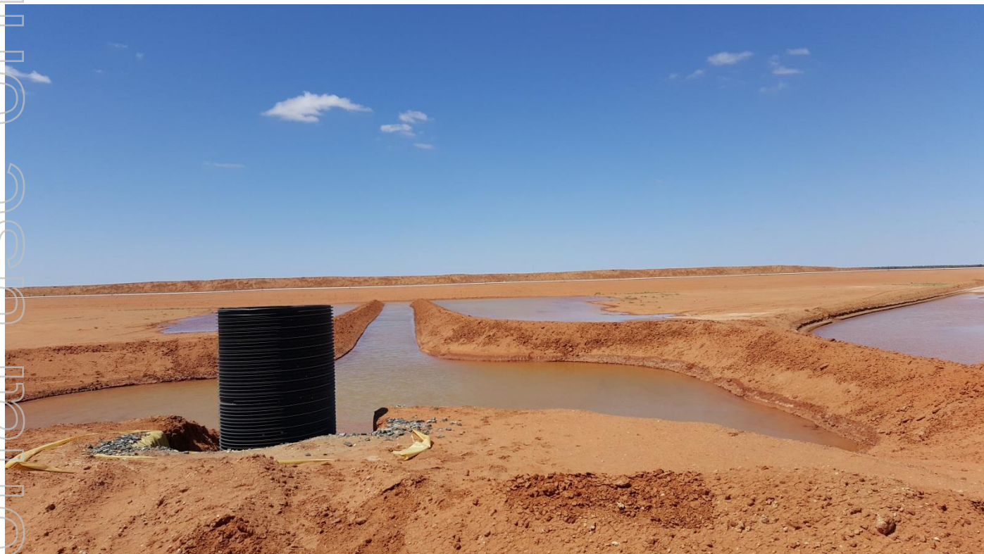
Tailings storage facility containing groundwater dewatered from the open pit
