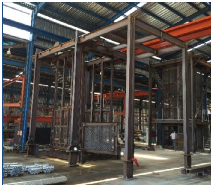
Photo 3. Headframe trial assembly - base section
