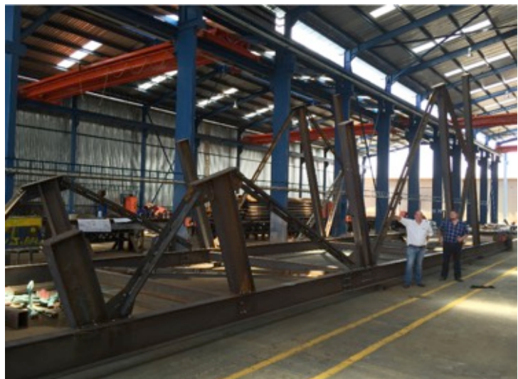
Photo 6. Headframe trial assembly - raker legs
