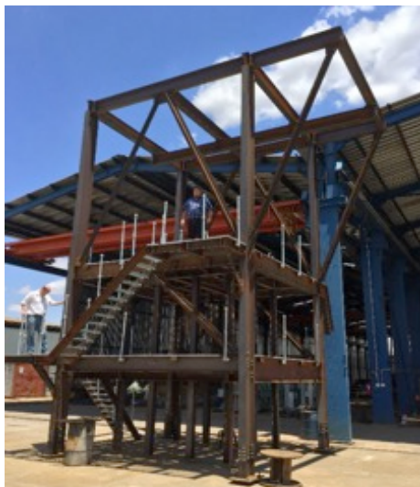
Photo 5. Headframe trial assembly - top section
