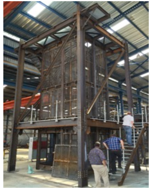
Photo 4. Headframe trial assembly - mid-section
