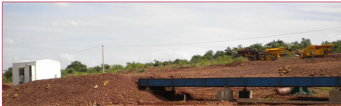
NSL Stockyard facilities, including weighbridge
