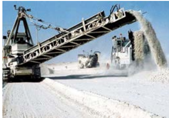
Wirtgen Surface Miner Cutting Salt
