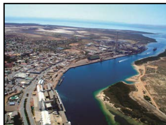
Figure 1 Aerial view of Port Pirie
