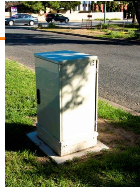
Fibre Distributing Hub
