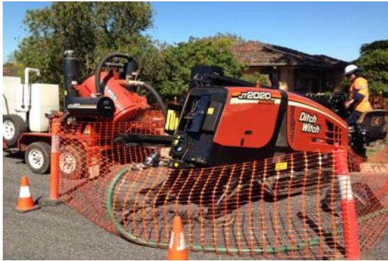
Vac truck assisting in pit clearing
