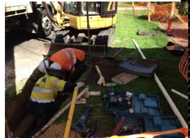
Trench cutting prior to laying new conduit
