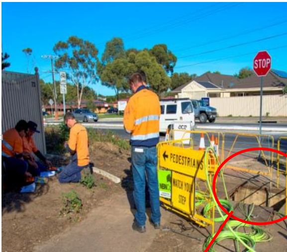
Open pit with fibre cable hauled through it
