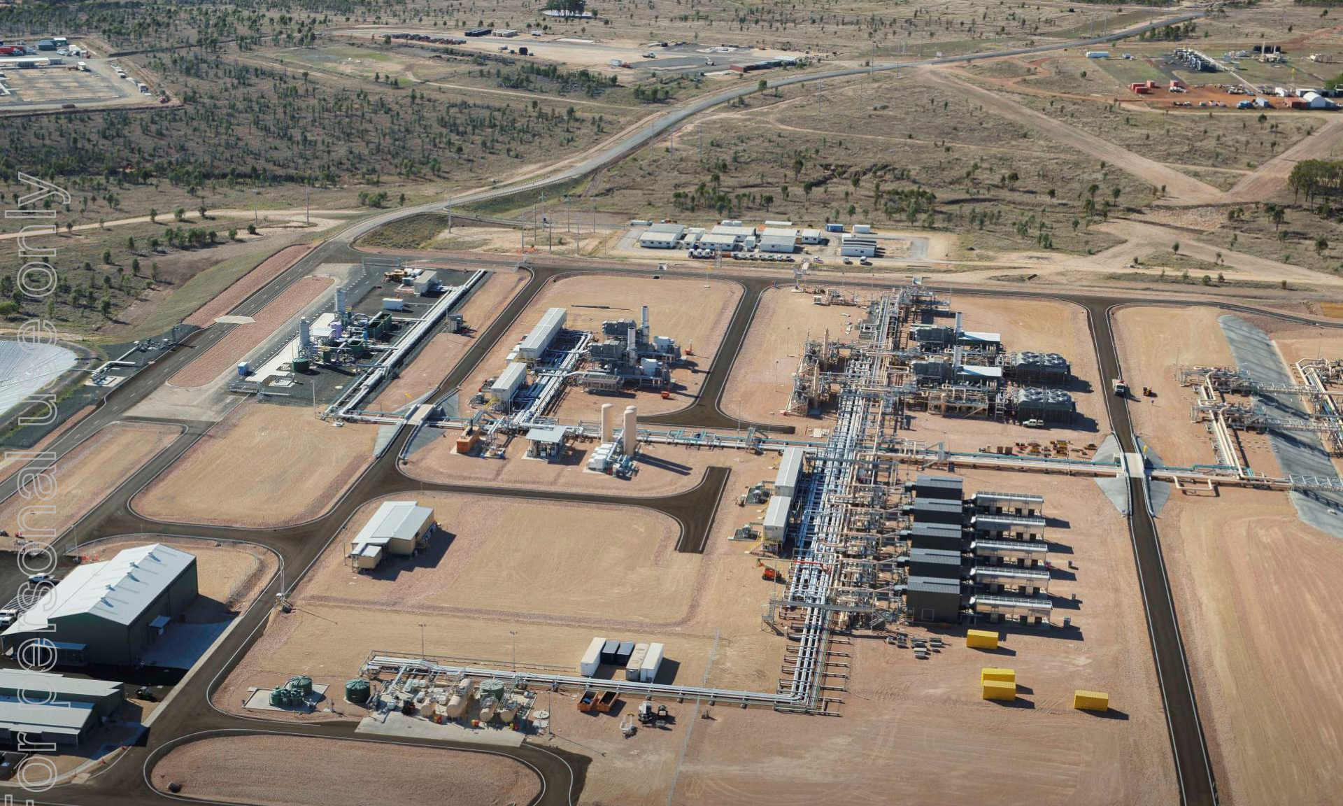
Fairview Hub 5 160 TJ/day capacity - construction and commissioning complete
