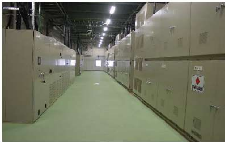
Figure 6 – VRB cell stacks at Tomamae Wind Farm (Source: J-Power)
