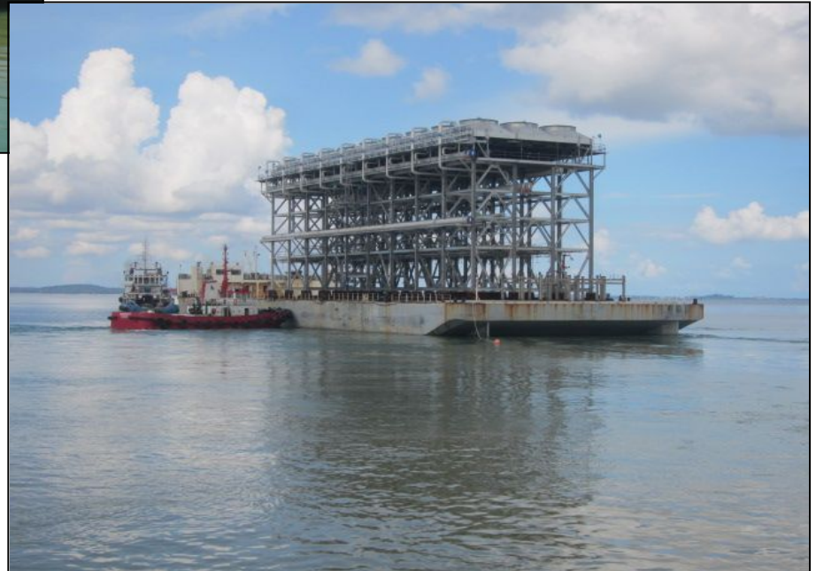
Propane Condenser 202ND shipped 13 May
