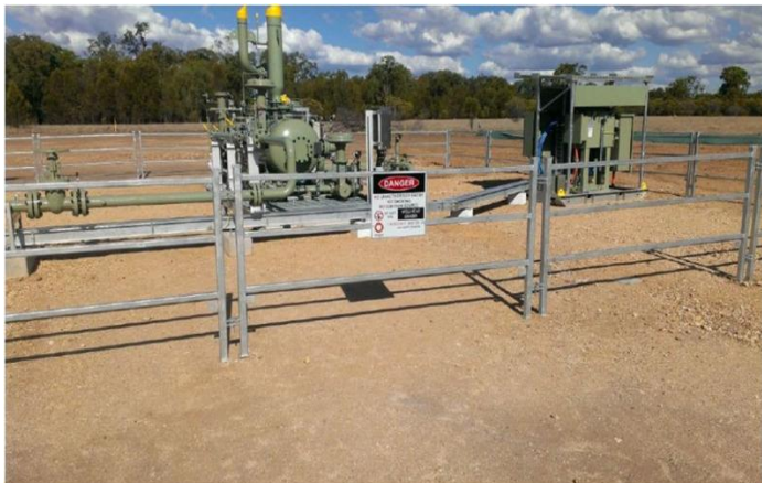
Orana completed Wellhead Separator Installation
