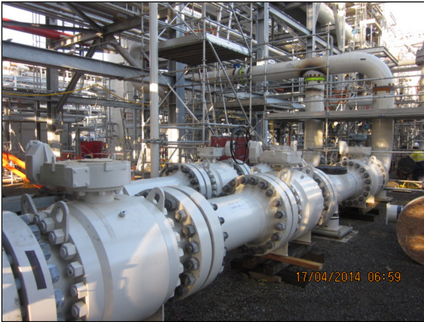
Hot Oil Heater/Incinerator Area - Piping Installation
