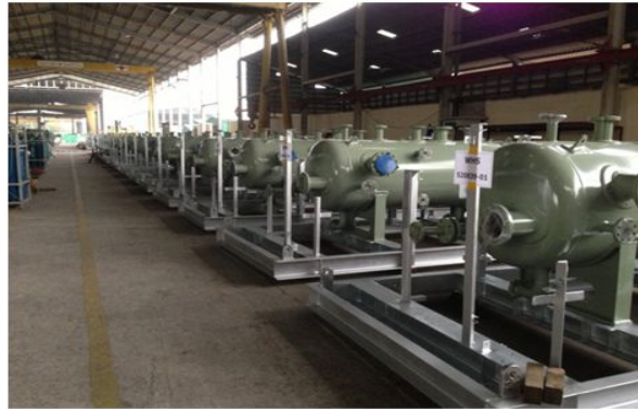
WHS SHIPMENT 23, 12 Vessels Mounted on Skids, Pipe Fit Ups Commenced
