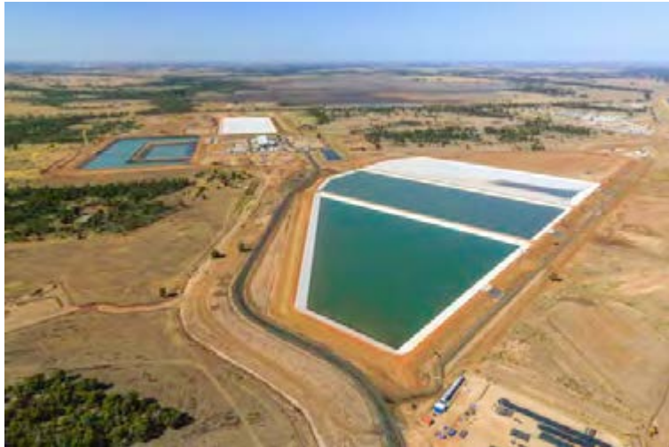
Condabri Central - water and brine ponds, February 2014
