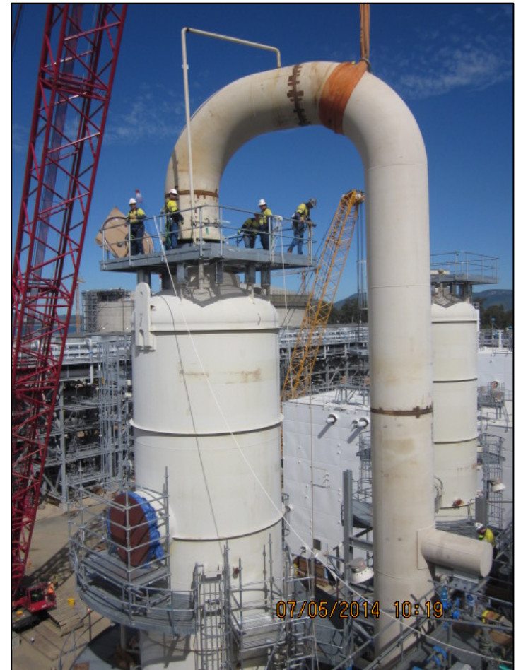
Propane Refrigeration Area - Setting "Candy Cane" on Propane Suction Drum
