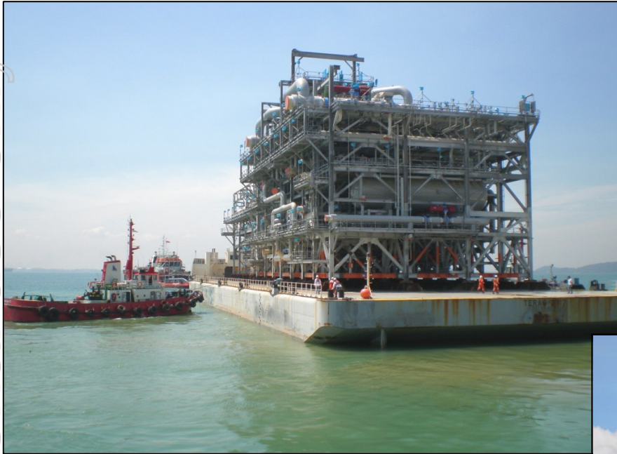
Final Train 1 Module (Propane Chiller 101JA) & First Train 2 Module (Sub-Cooler 202 NE) shipped on 22 April
