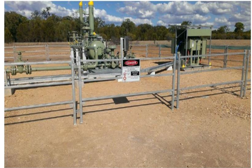
Orana completed Wellhead Separator Installation
