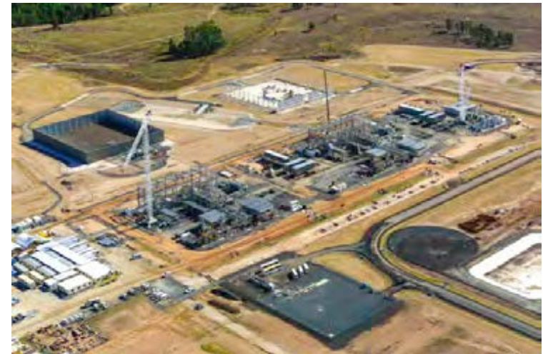
Orana - Gas Processing Facility
