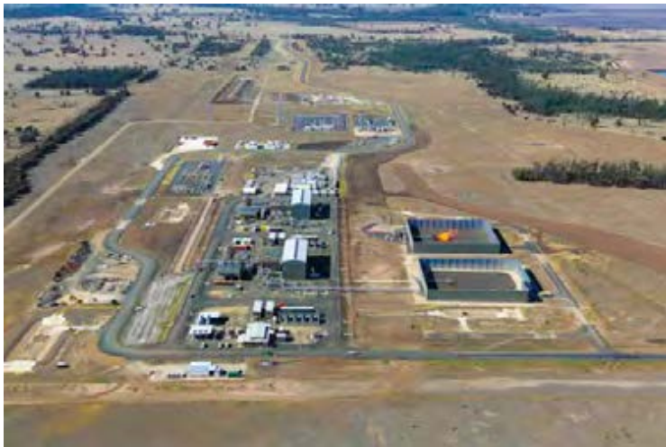
Condabri Central - Gas Processing Facility
