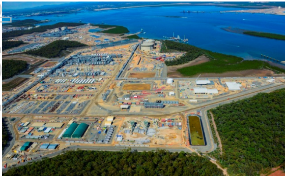
Curtis Island site, May 2014
