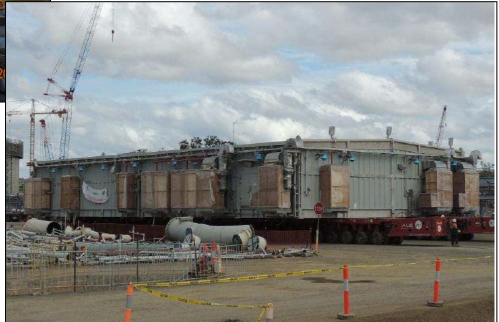
Compressor Substation being moved into position
