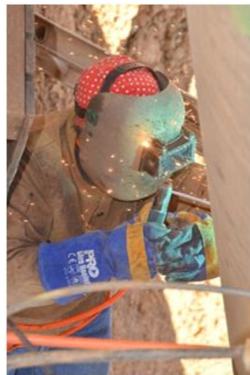
Last Golden Weld on the Main Transmission Pipeline
