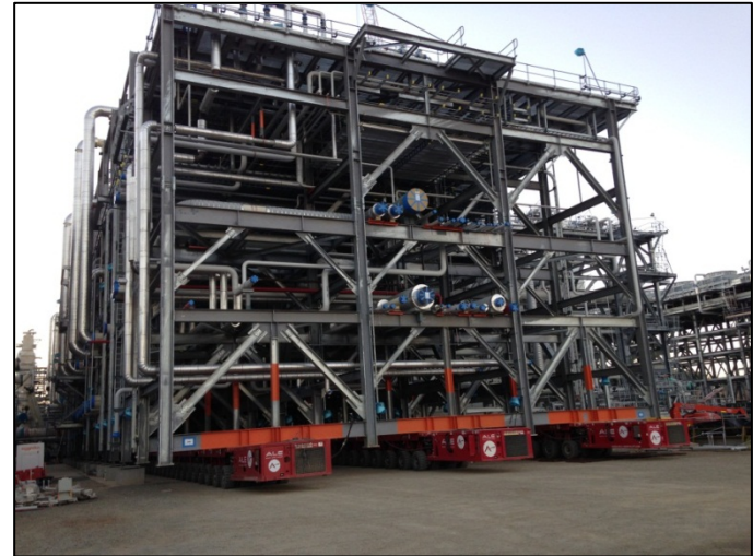
Module 101DA delivered to site
