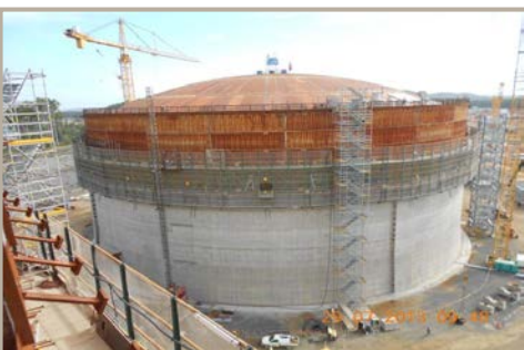
Downstream Project 45% Complete 1
