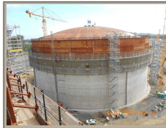
LNG Tank B - roof raised on 29 July
