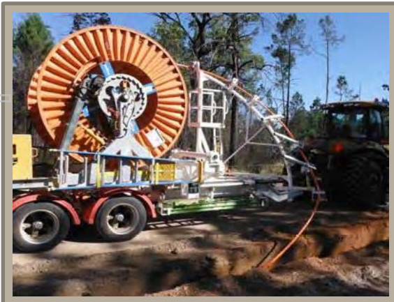
Cable installation in Combabula
