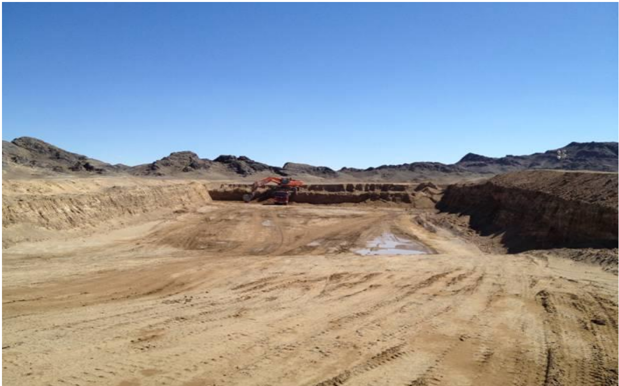
This photograph shows the test pit at depth of approximately 5 metres, with about 3 metres of overburden on top of coal still to be excavated.
