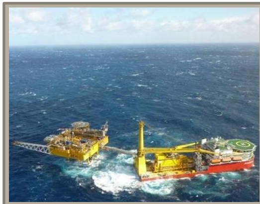
Jascon 25 construction vessel at Yolla
