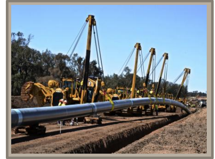
Laying of pipe
