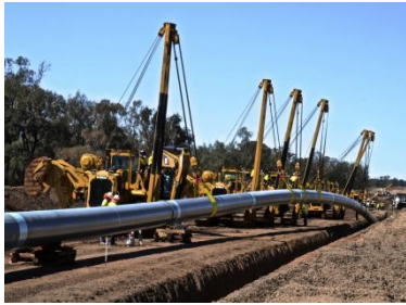
Upstream Project 29% Complete
