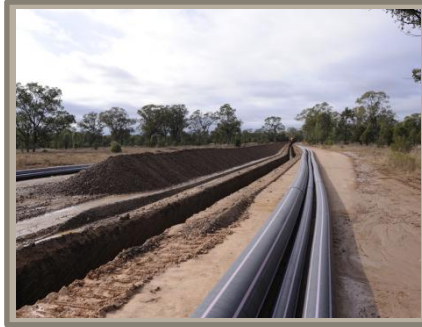
Laying of gathering pipe
