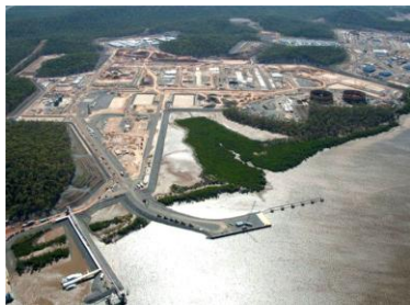
Downstream Project 31% Complete
