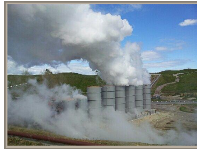
Steam Field 2 Dump Station (Te Mihi) being used for the first time
