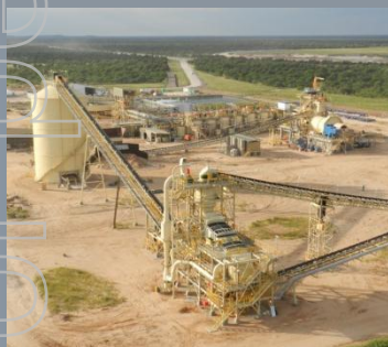
Screen plant and crushed ore bin
