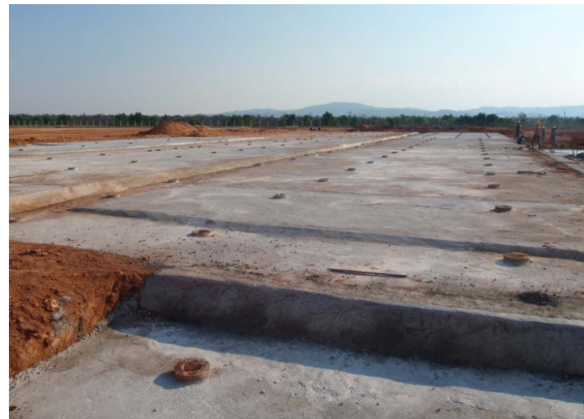
Blinding slab being prepared for concrete
