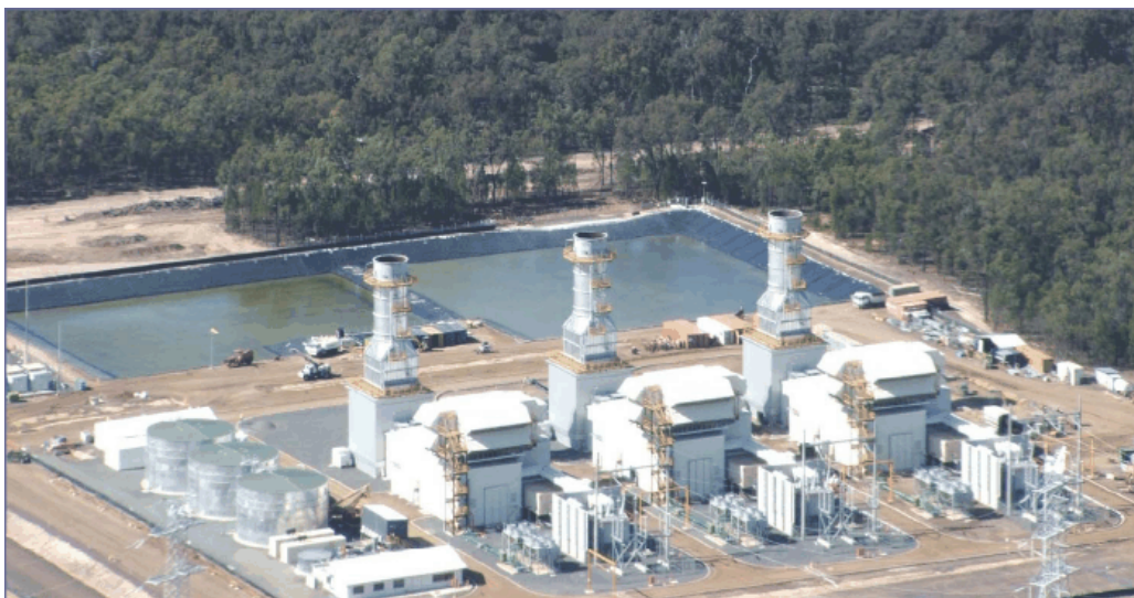
Braemar 2 Power Station – three 150 MW Siemens Gas Turbines
