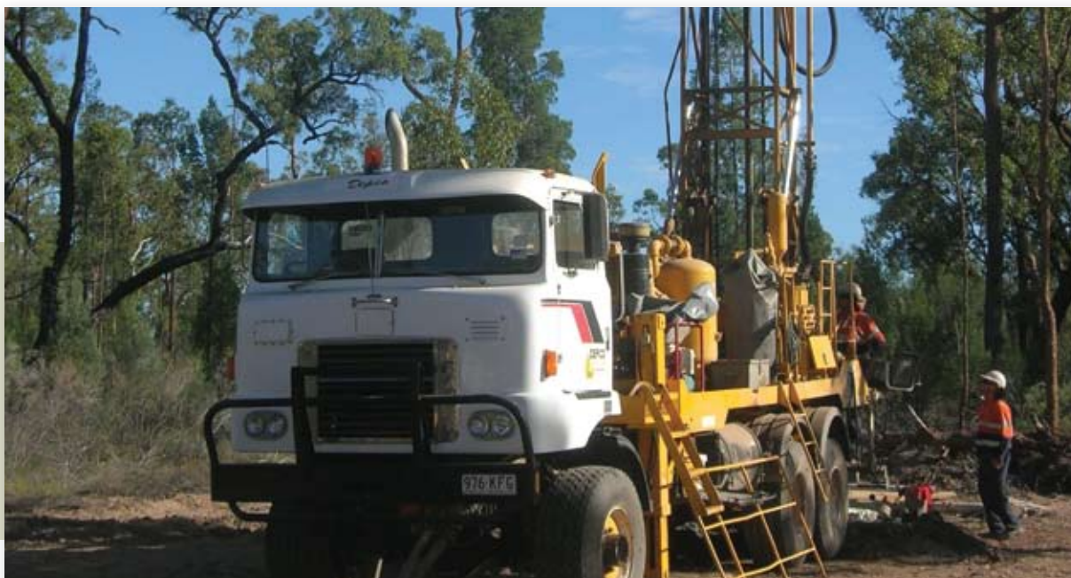
Drilling at the Surat Project
