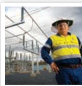
QGC will sell electricity from its Condamine Power Station to the National Electricity Market through the Columboola Switching Station, where contractor i.Power Solutions' Trevor Scott is pictured.
