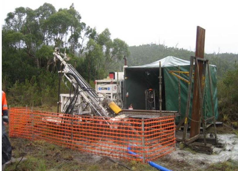
Drilling hole LV001 at Stanley River
