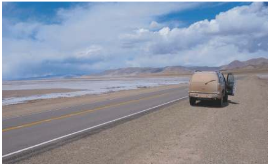
Olaroz - Sealed road access with buried gas pipeline
