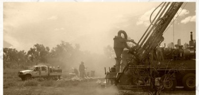
RC drill rig and support crew
