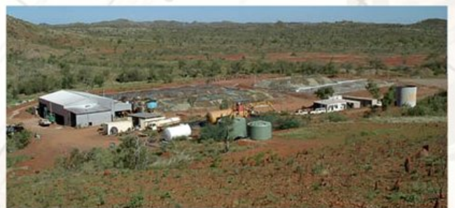
Mt Norma plant and leach pads
