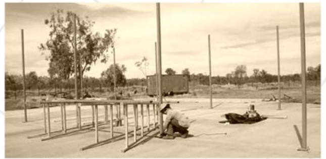
New 1,000m 2 diamond core storage facility under construction
