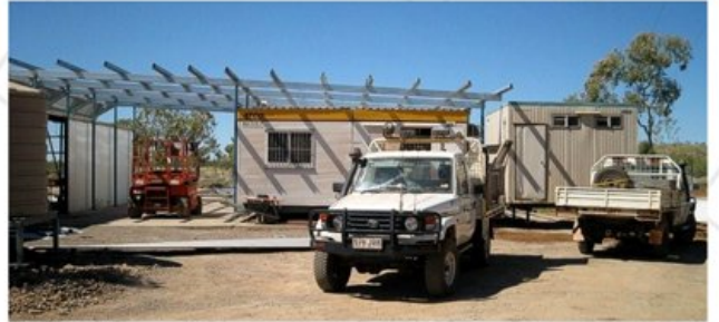
Lab under construction
