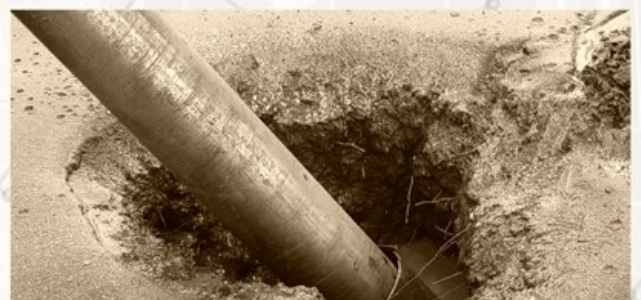
Diamond drill with copper filings evident in wash-back
