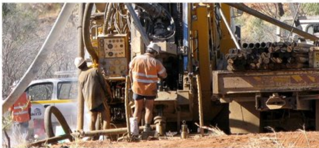
RC drill rig and crew at work
