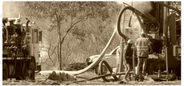
RC drill crew at work
