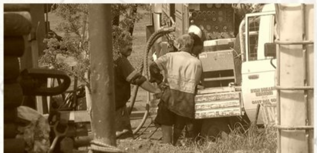
RC rig at work
