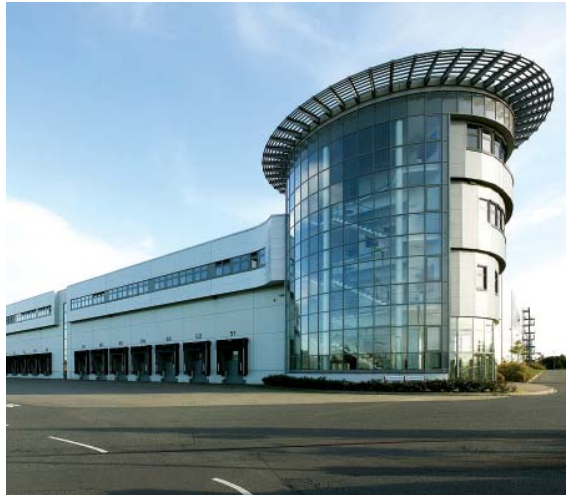
BRIESELANG DISTRIBUTION CENTRE BRIESELANG, GERMANY
