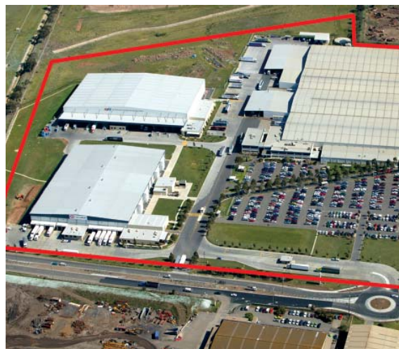
LAVERTON DISTRIBUTION CENTRE LAVERTON, VICTORIA AUSTRALIA
