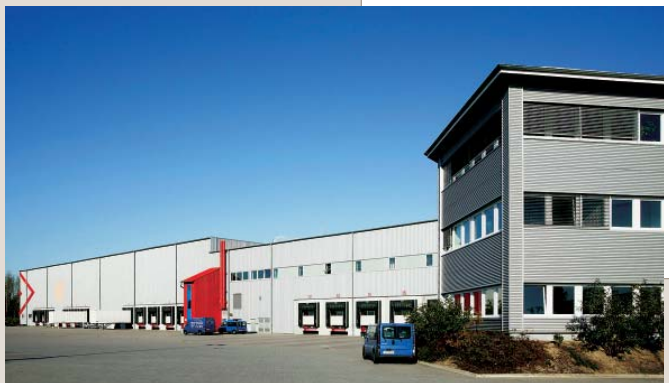
BRIESELANG DISTRIBUTION CENTRE, BRIESELANG, GERMANY
