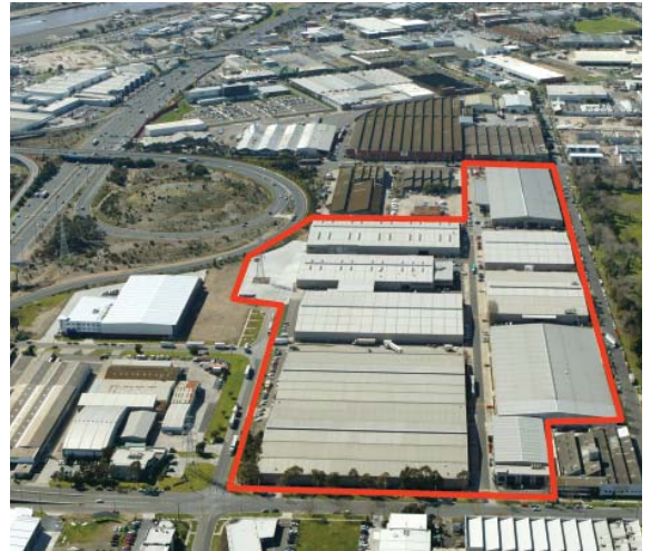
PORT MELBOURNE INDUSTRIAL ESTATE PORT MELBOURNE, VICTORIA AUSTRALIA
