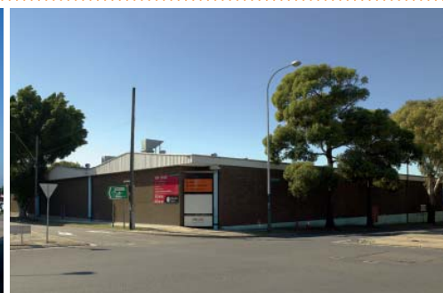
EUSTON BUSINESS CENTRE, NSW, AUSTRALIA
